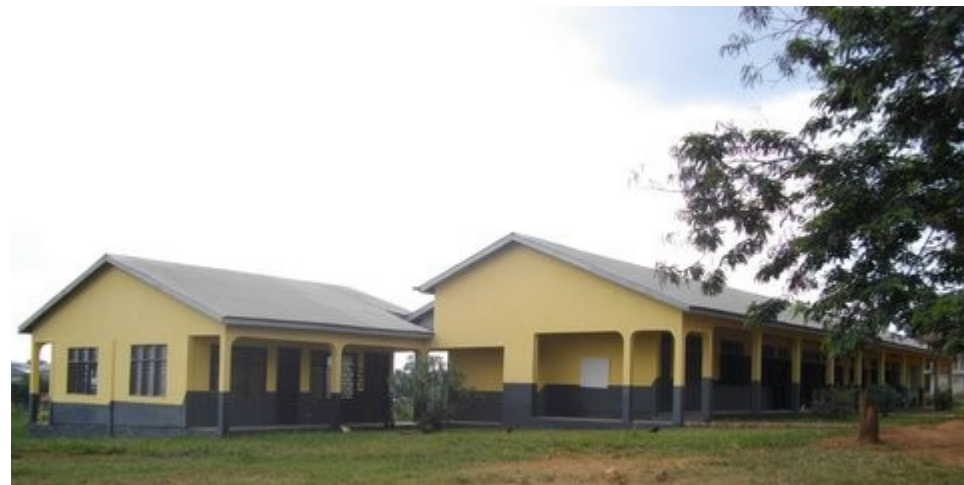
← The newly painted Senior High School at Adumasa
